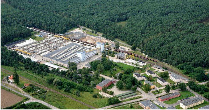
Prestressed Concrete Sleepers Manufacture
