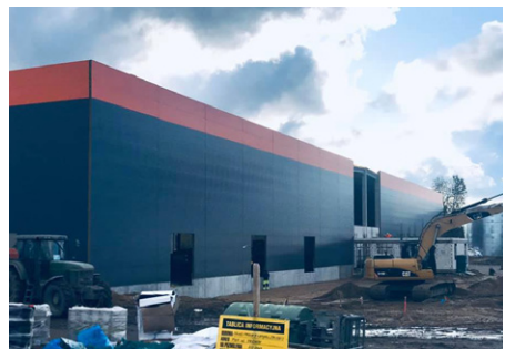
Construction works of the "Zbyszko Company" plant in Piła
