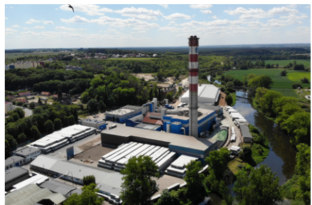
Ardagh Glass S.A. plant – the Ujście commune
